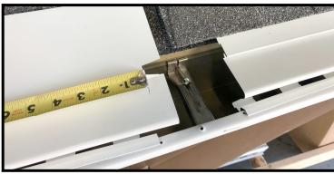
Mark the nose of the panel for your length, and using a roofing square, mark the panel at a 45 degree angle for trimming. The front lip screw rail will need to be trimmed by about an additional 1" – 1-1/2" as shown.
