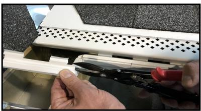
Next, trim the screw-tabs from the right end of the left side panel, then mark the nose of the panel 2-1/2" from the right end. Then mark the lip of the panel at 3".
