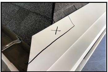
Place the panel in place under the first row of shingles, interlocking the right side tabs with the previous panel, and attach to the gutter using 3 zipscrews.
