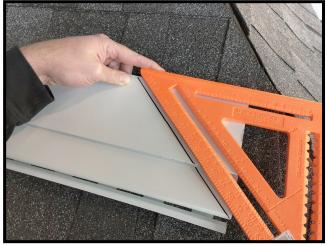
Trim the 45-degree angle and about 1-1/2" of the front screw rail as shown.
