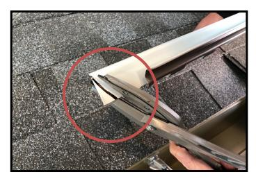
The panel may need to also be trimmed as shown to allow clearance for the ridge cap nails.
