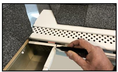
Remove the panel and trim the front lip and tabs from the edge of the panel as shown. Replace the panel and use 3 zipscrews to attach the panel to the lip of the gutter.
