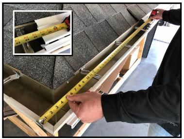
Measure from the right end of the panel to be installed, BUT not including the screw tab, as shown.
